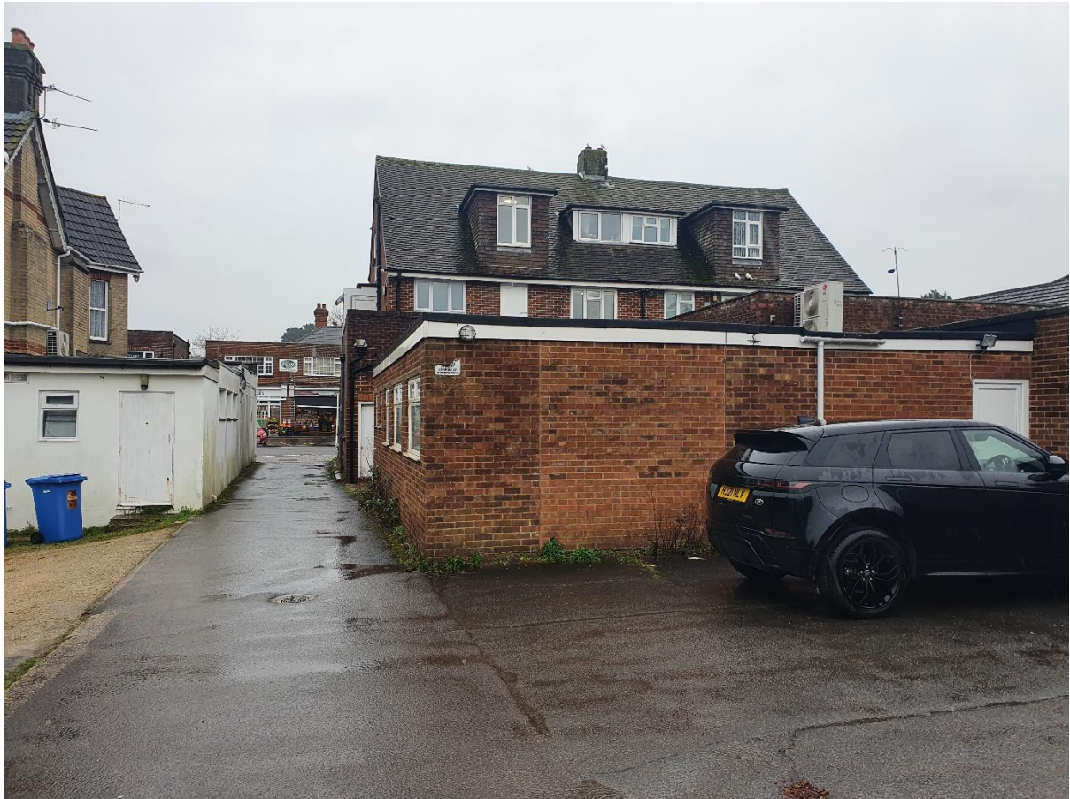
189 Lower Blandford Rd site visit photos 16/03/2022
